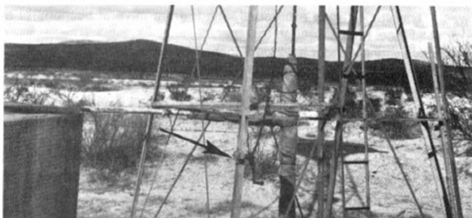
Windmill. Note windlass (arrow).
